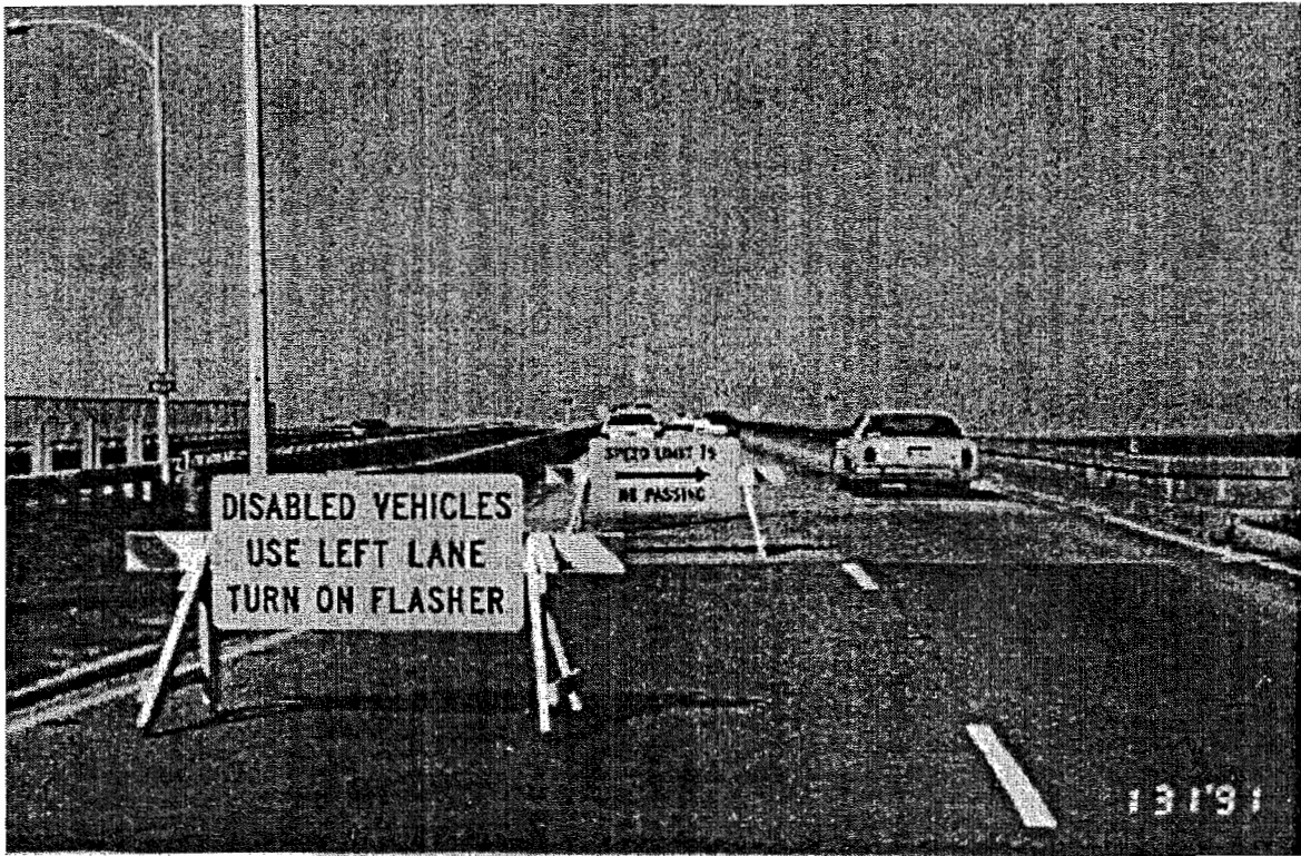
Figure 7. Fog abatement sign configuration illustrates the view from ground level to what motorists would encounter when controls have been put in place on the bridge.
